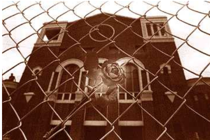
A rose stuck in the fence outside Immaculate Conception Church is all that remains of a 1981 protest vigil as workers continue to dismantle the Poletown landmark.
